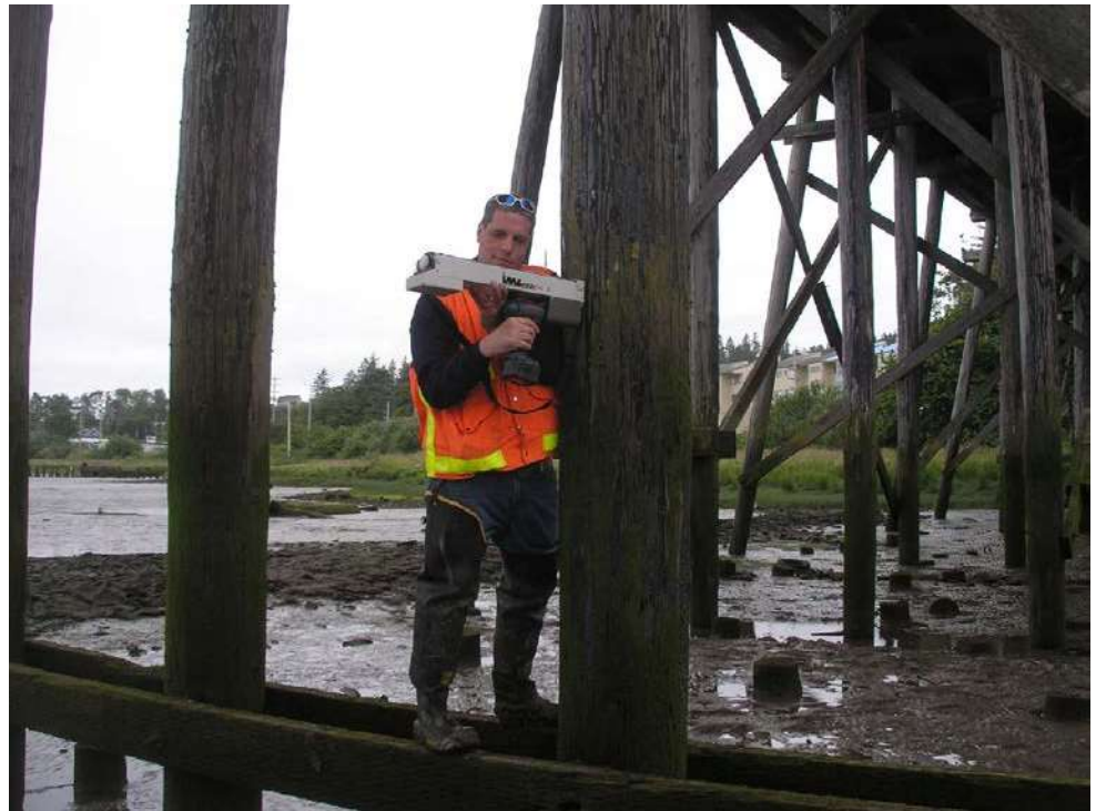
Figure 15.1.6 Inspector Using Decay Detection Device
