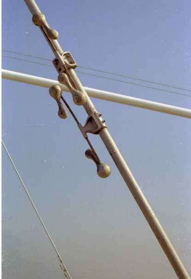
Figure 16.1.51 Tuned Mass Damper System
