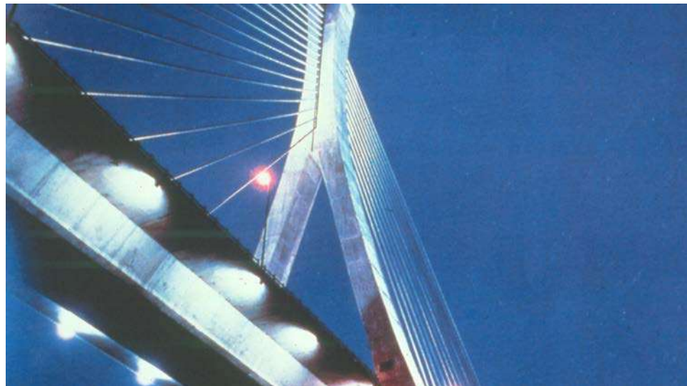
Figure 16.1.29 Single Vertical Plane Cable System
