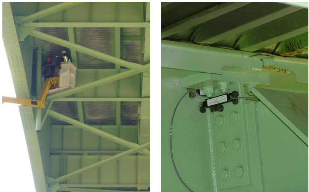
Figure 15.4.1 Installation of Sensors
