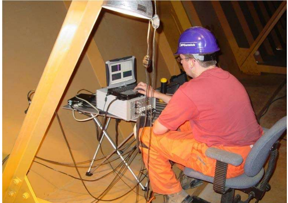
Figure 15.3.2 Inspector Using Acoustic Emissions to Determine Crack Propagation
