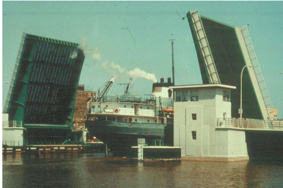
Figure 16.2.9 Double-Leaf Rolling Lift Bascule
