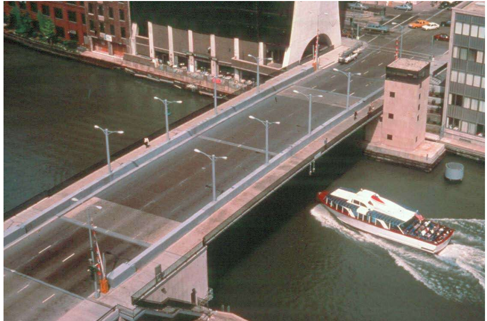
Figure 16.2.11 Double-Leaf Trunnion Bascule Bridge
