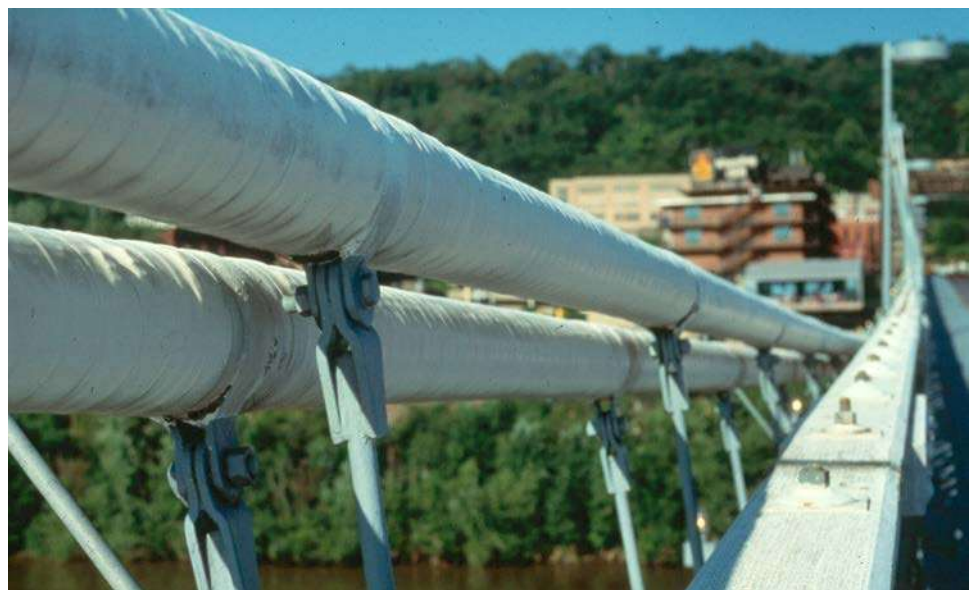
Figure 16.1.12 Cable Wrapping on the Wheeling Suspension Bridge
