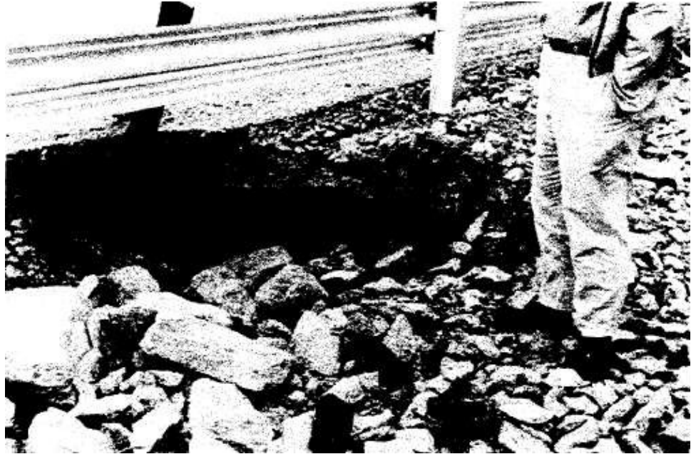
Figure 14.3.10 (Exhibit 68) Surface Hole Above Open Joint
