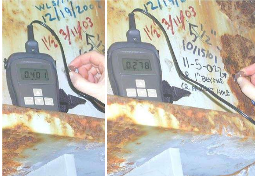
Figure 15.3.9 Ultrasonic Thickness Depth Meter (D-meter)
