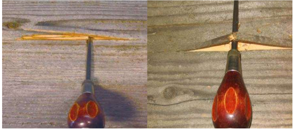
Figure 15.1.8 Pick Test: Sound Wood, Decayed Wood
