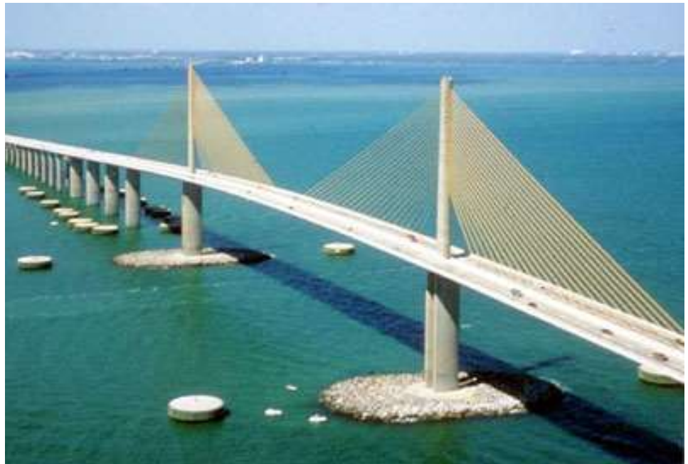
Figure 16.1.4 Sunshine Skyway Cable-Stayed Bridge in Tampa Bay, Florida
