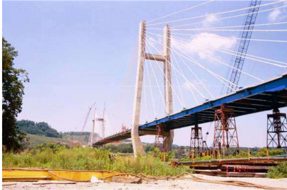
Figure 16.1.2 Maysville Cable-Stay Bridge
