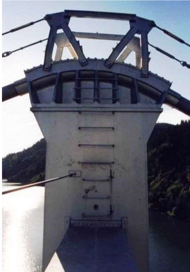
Figure 16.1.32 Cable Saddle
