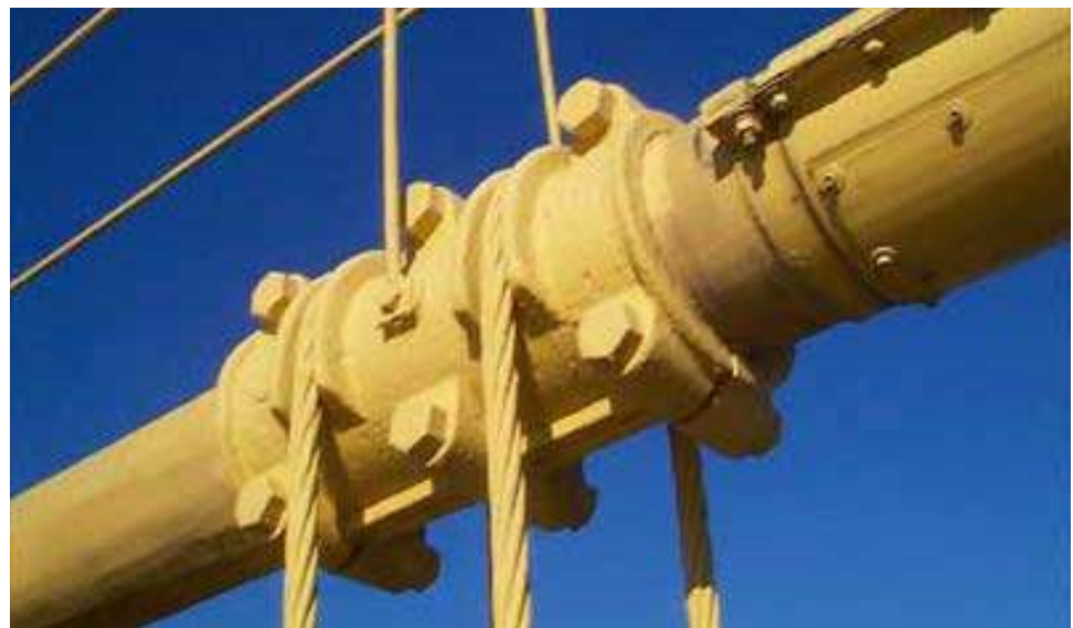
Figure 16.1.19 Grooved Cable Bands
