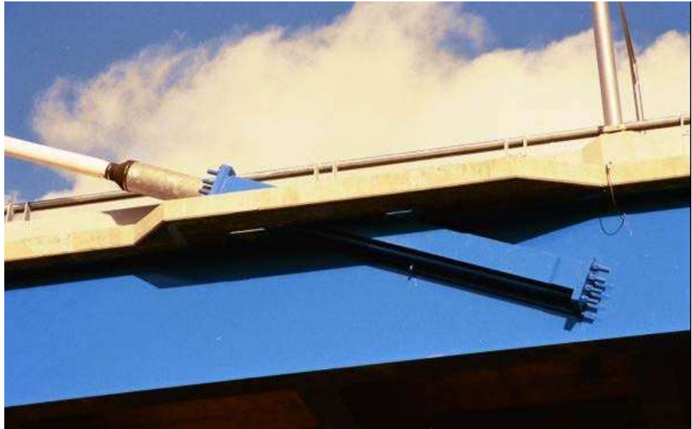
Figure 16.1.33 Cable Deck Anchorage
