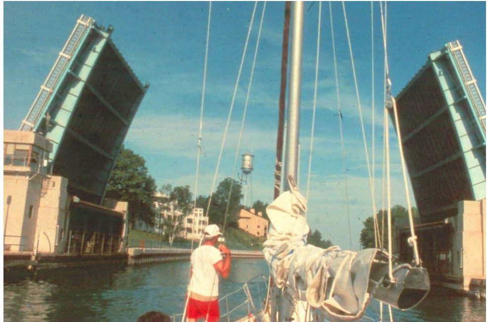
Figure 16.2.7 Bascule Bridge in the Open Position
