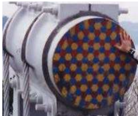
Figure 16.1.8 Parallel Strand Cable
