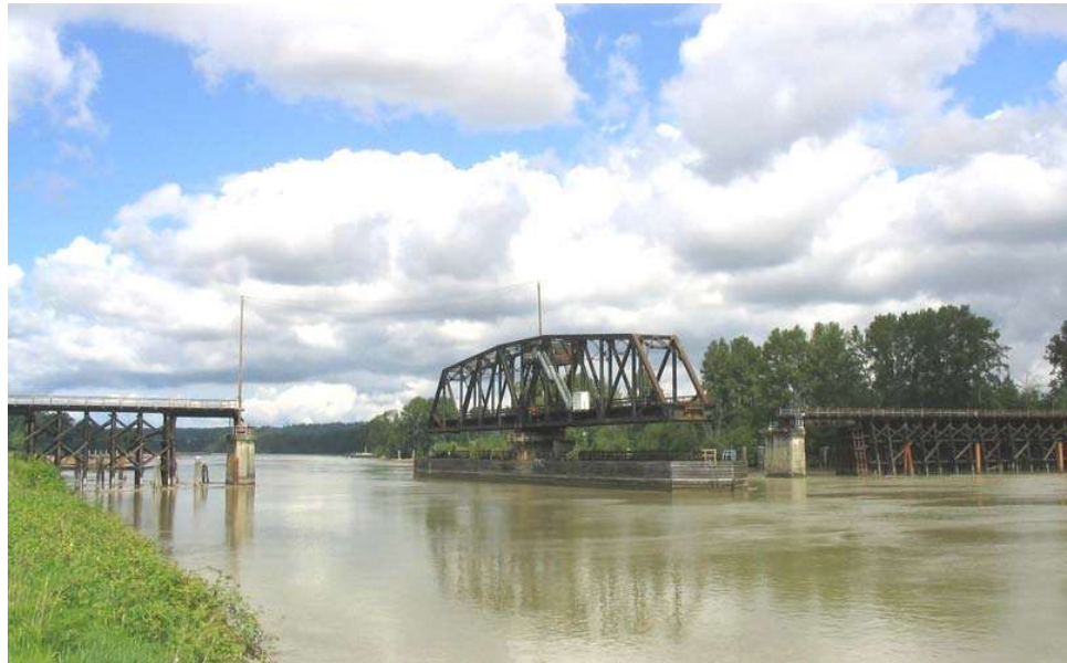
Figure 16.2.4 Center-Bearing Swing Bridge
