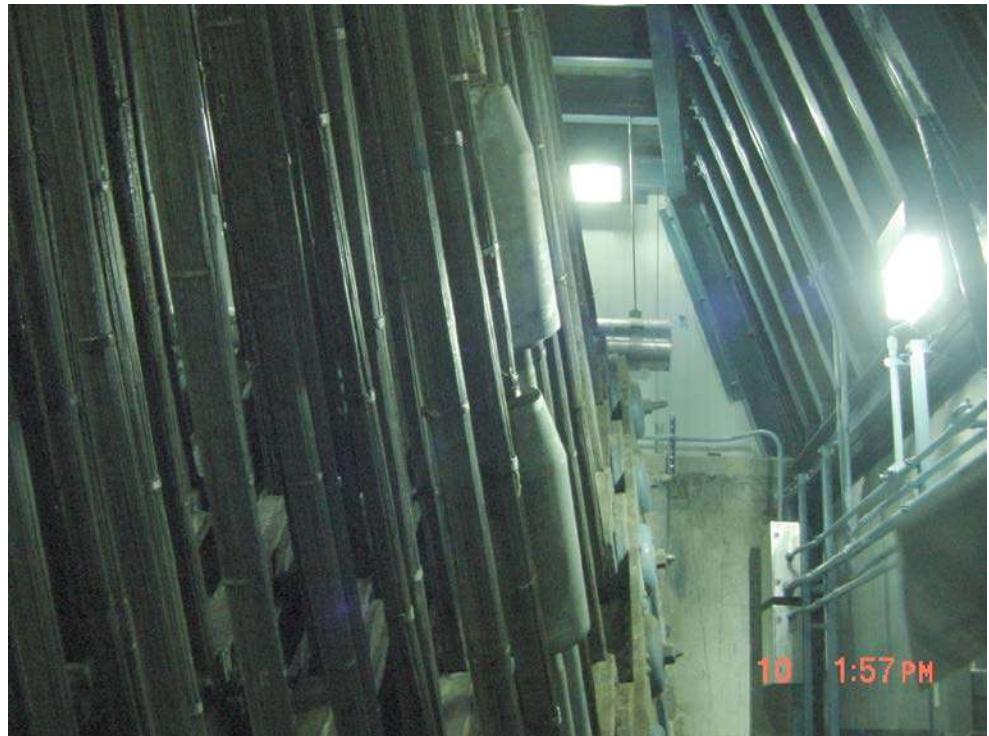
Figure 16.1.37 Anchorage Interior of Ben Franklin Bridge, Philadelphia, PA
