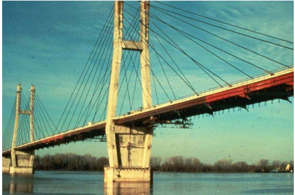
Figure 16.1.30 Double Vertical Plane Cable System
