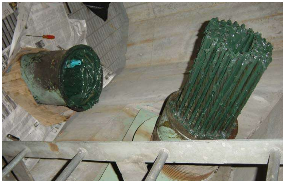
Figure 16.1.34 Anchor Inspection on Veterans Bridge
