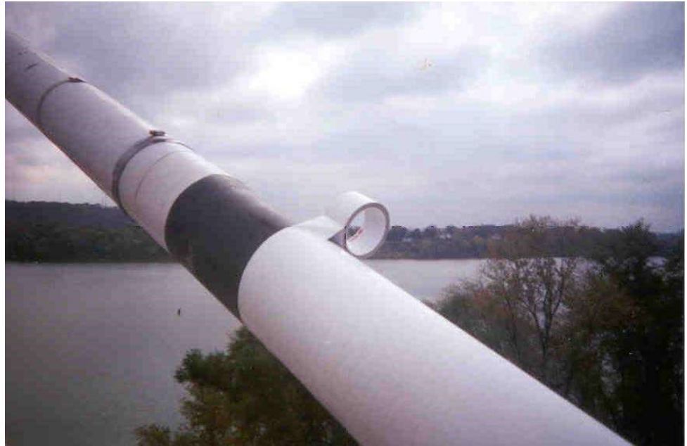
Figure 16.1.42 Cable Wrapping Placement
