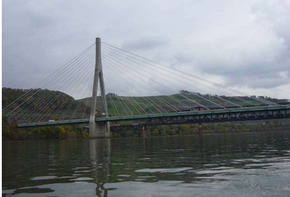
Figure 16.1.41 Cable-Stayed Bridge Cables
