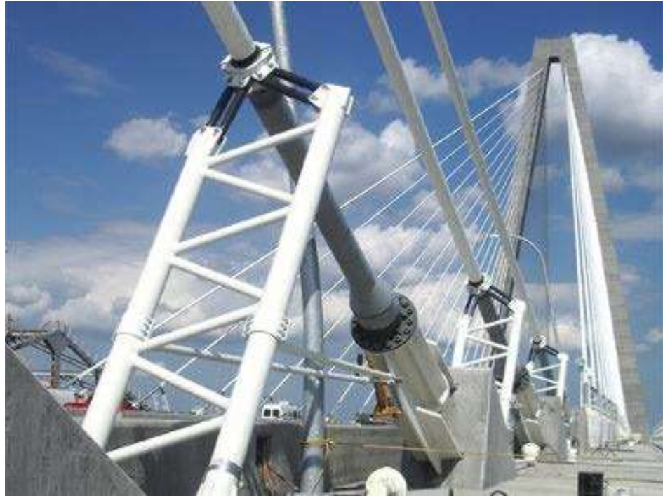
Figure 16.1.48 Shock Absorber Damper System
